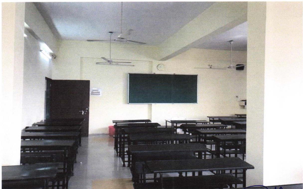
15. FIFTH FLOOR ROOM NO. 74
