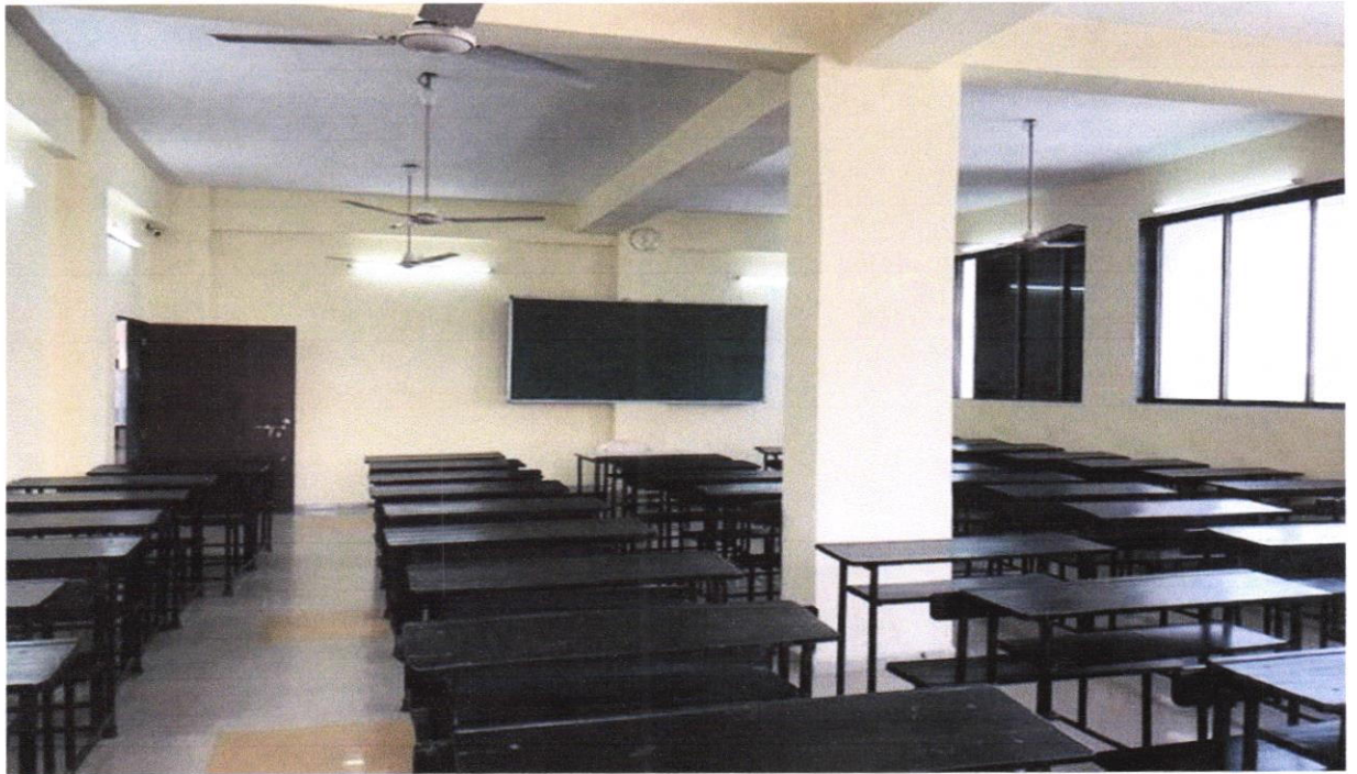
18. FIFTH FLOOR ROOM NO. 66
